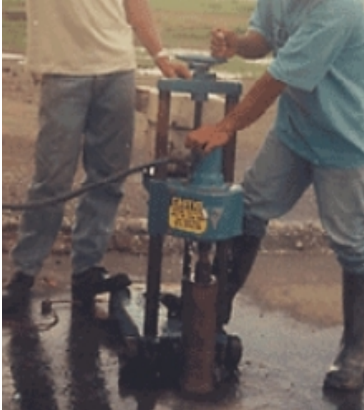
Coring of Asphalt Pavement. PGAI also has four (4) electric coring machines for coring of concrete structural elements in buildings and other structures.
